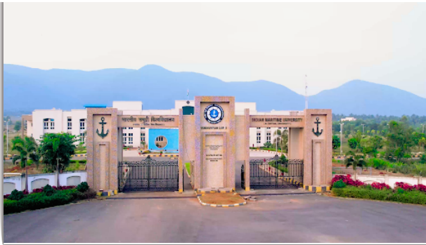
IMUV NEW CAMPUS, SABBAVARAM
