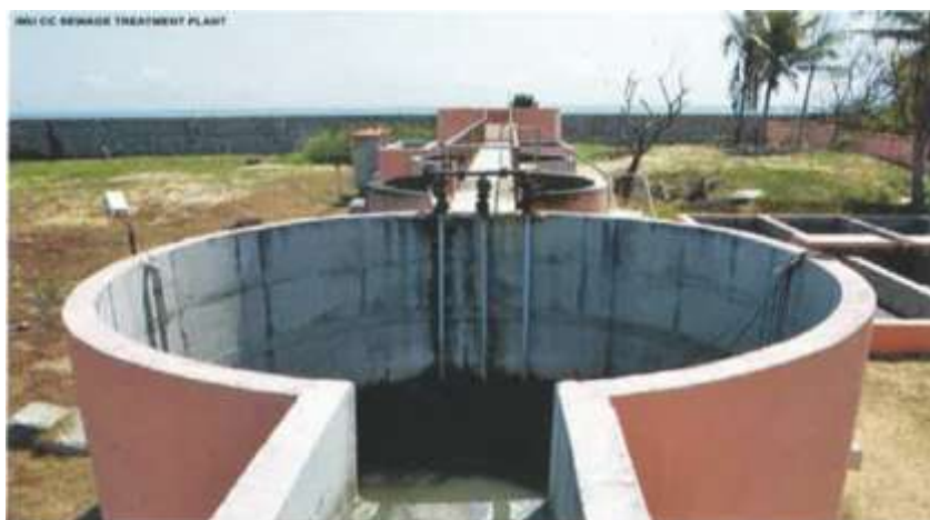
Sewage Treatment Plant
