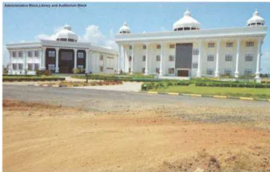
Administrative Block, Library and Auditorium Block
