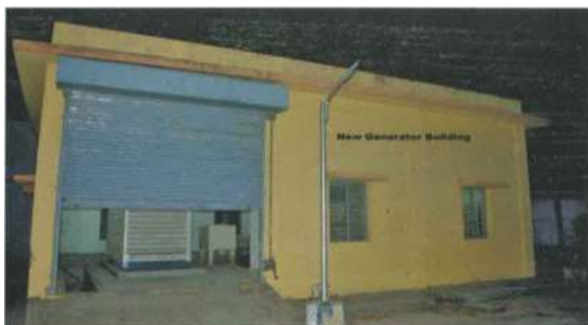
New Generator Building
